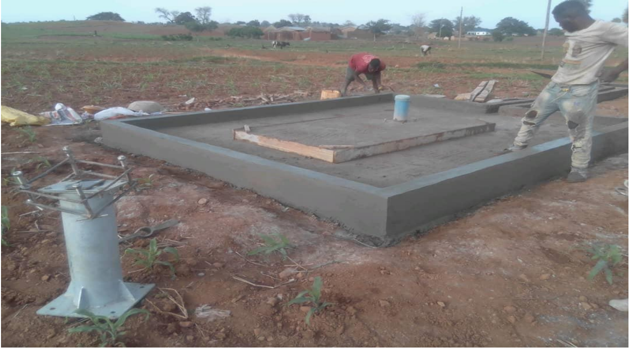
PLATFORM CONSTRUCTION AT KPATIA
