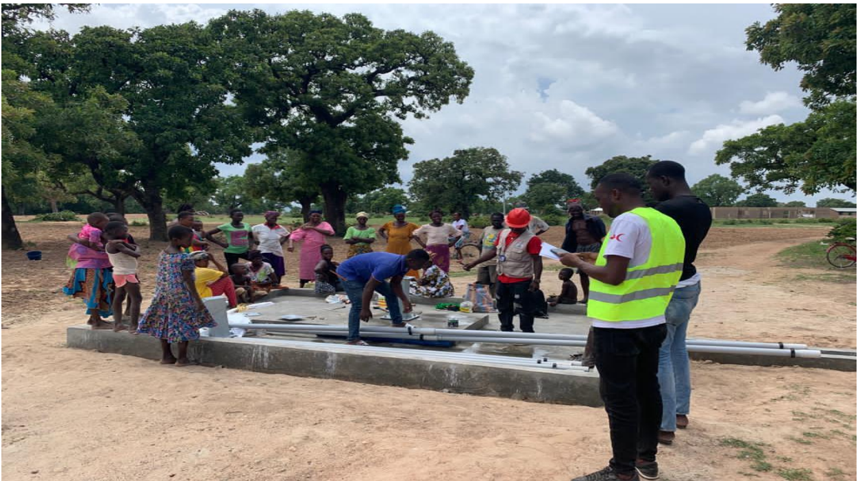
INSTALLATION OF PUMP AT MANYORO
