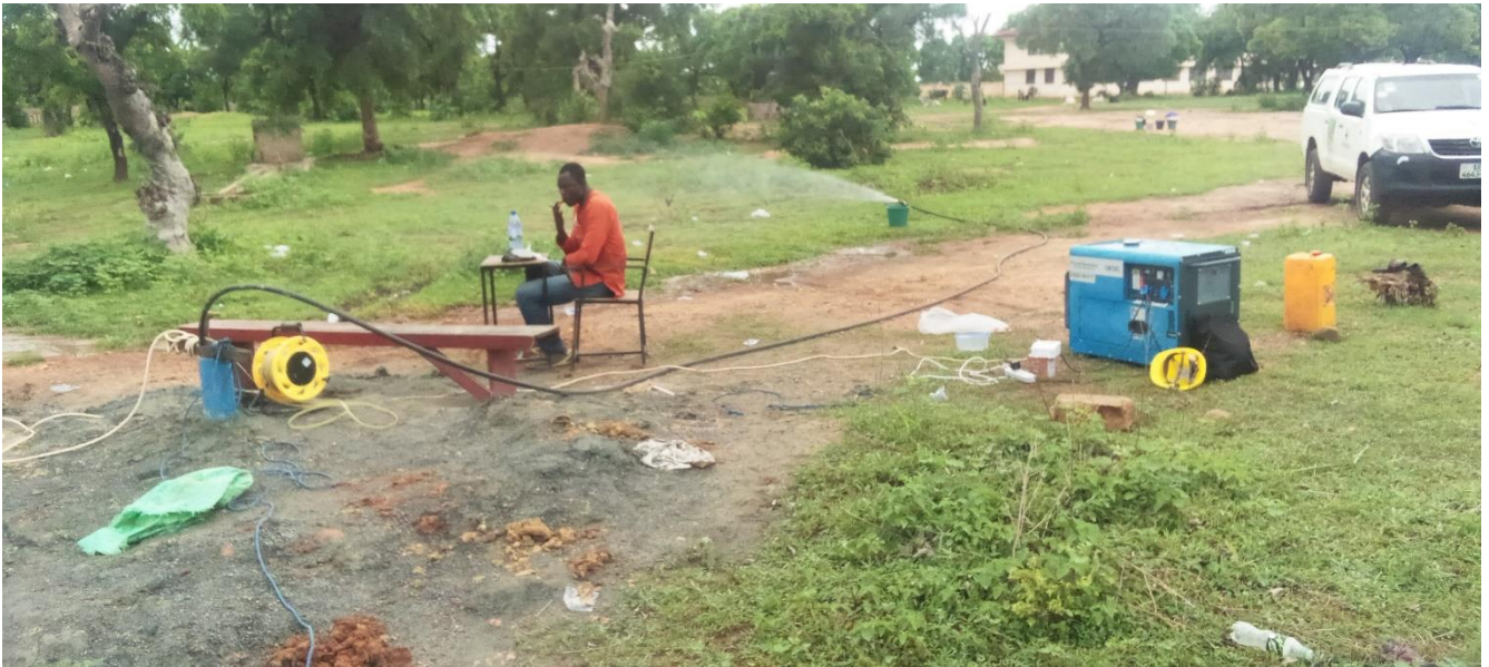
PUMPING TEST AT AWE SHTS
