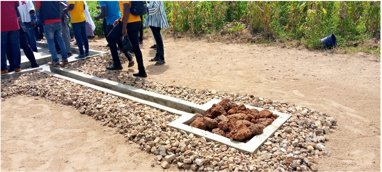
COMPLETE BOREHOLE AT LATEGA
