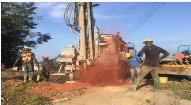
Drilling borehole in Kadewaso
