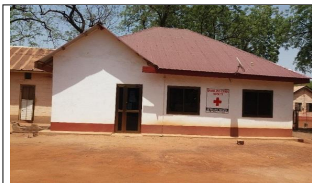
FRONT VIEW OF OFFICE
