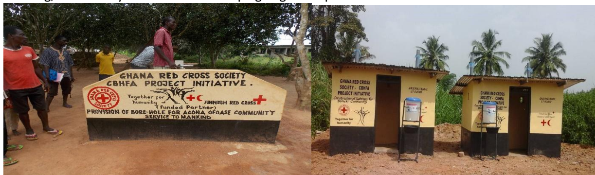
Picture of some of the boreholes and household toilets constructed under the CBHFA project
