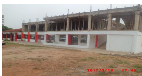
Current View: Work in Progress – National Headquarters, GRCS
