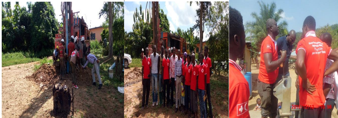
Drilling new Bore Holes and repairing existing but broken-down ones in the communities
