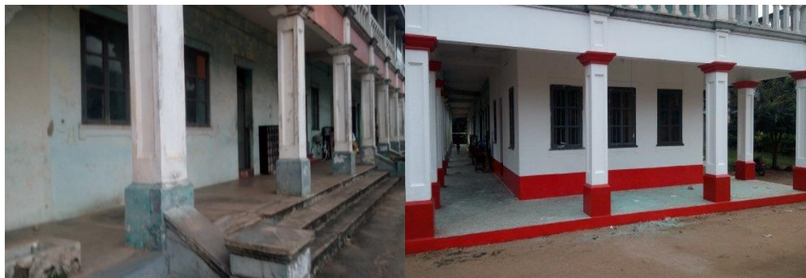
Before Renovation after Partial Completion of Renovation
