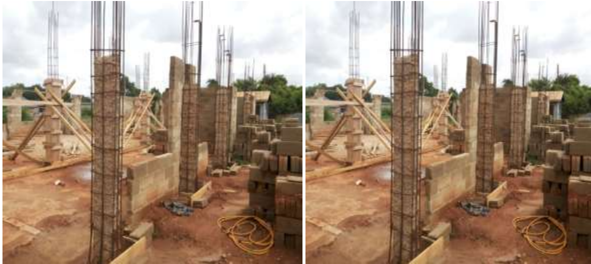
Pictures of the new site plan under construction.
