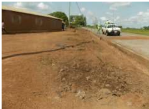
In picture is the de-silted drain in Baya, Brong Ahafo region.
