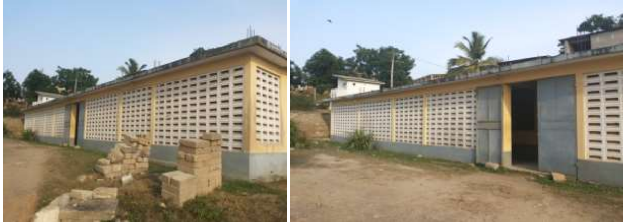
Hostel building in the Central Region ( Ground floor)
